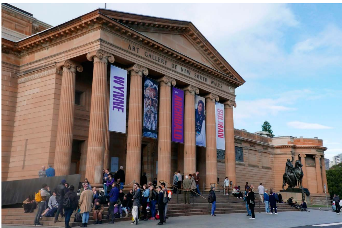
8. Art Gallery of New South Wales in Sydney – main entrance
