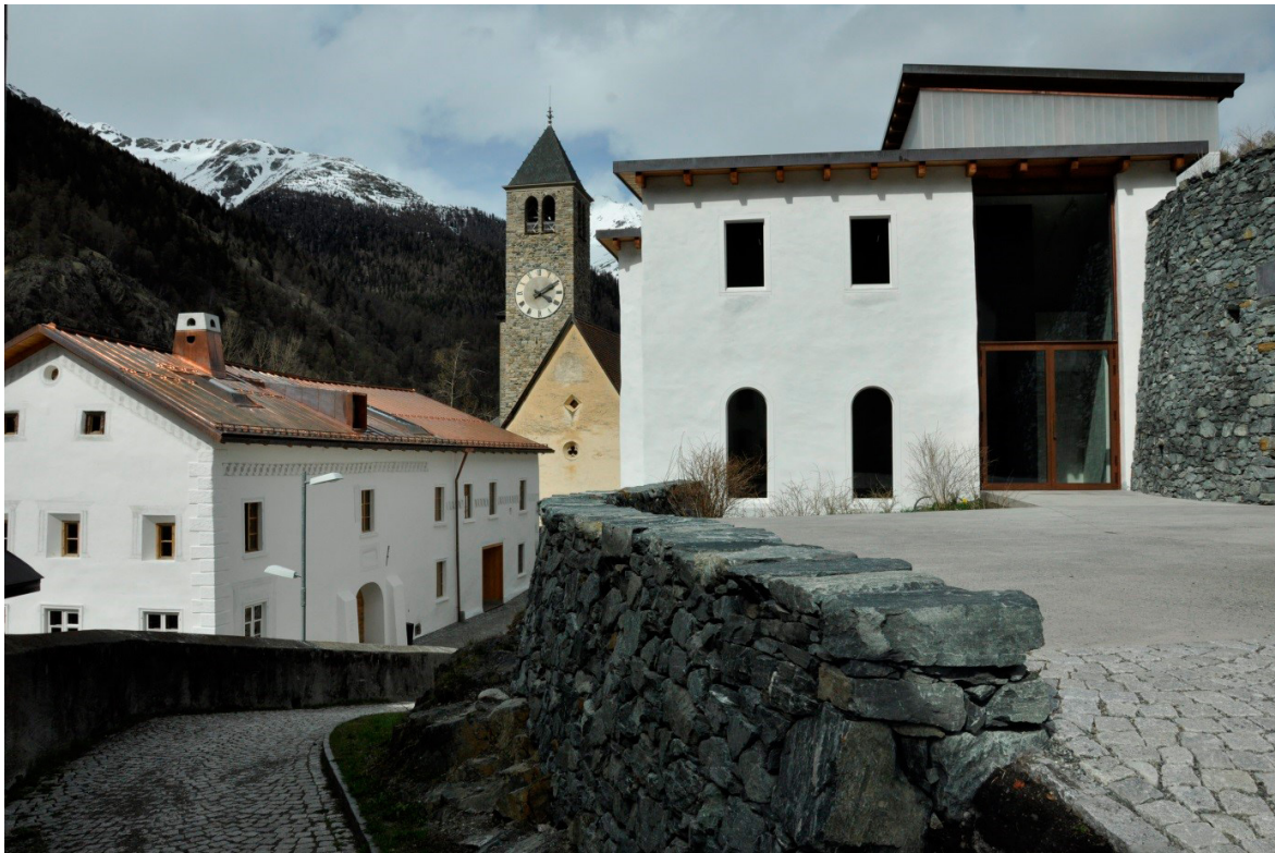
5. Muzeum Susch, new brewery building, Bieraria , in the foreground, housing the majority of display rooms, with a tower fan above
