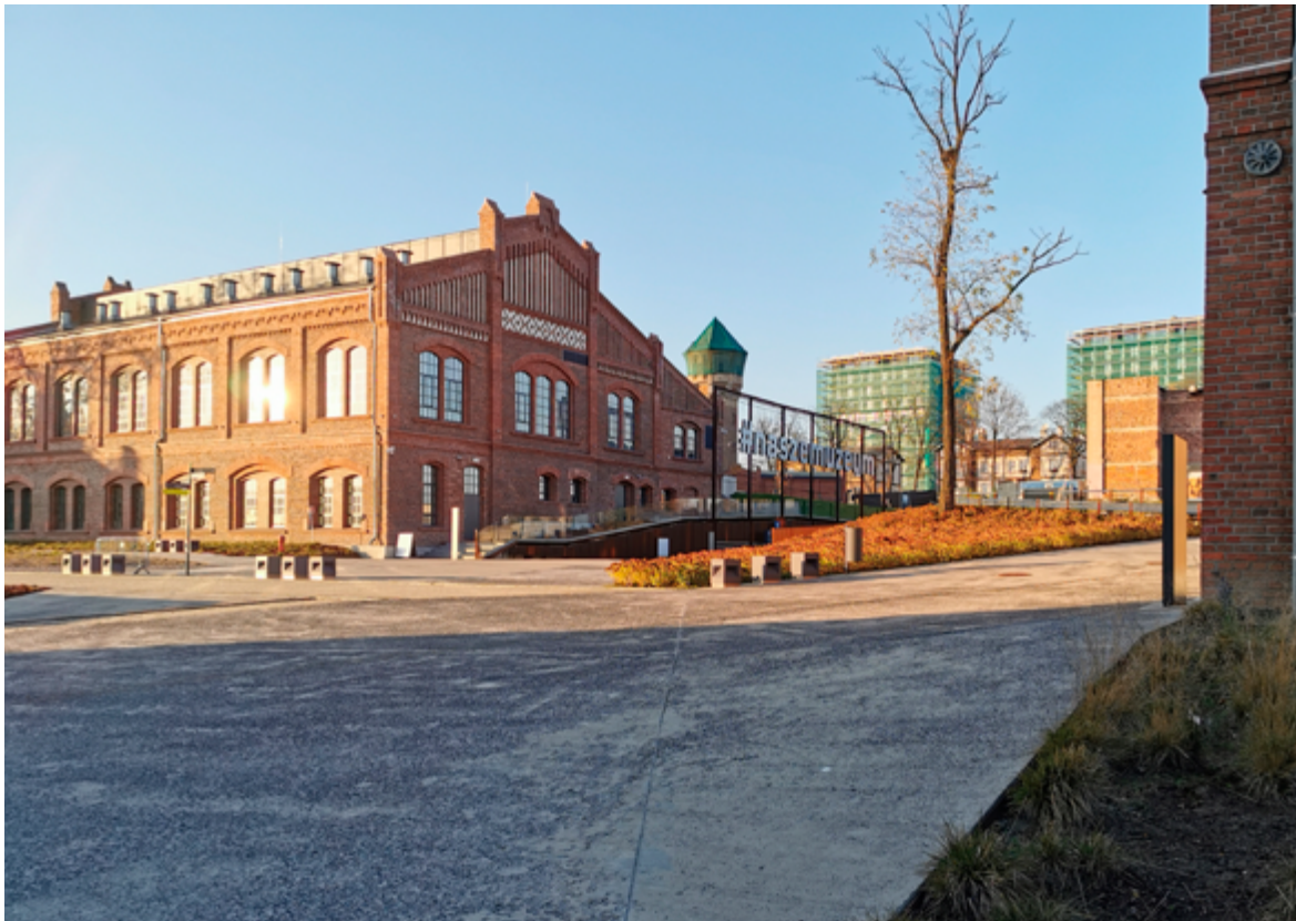
7. Building of a housing estate close behind the site of the Silesian Museum in Katowice, November 2020
